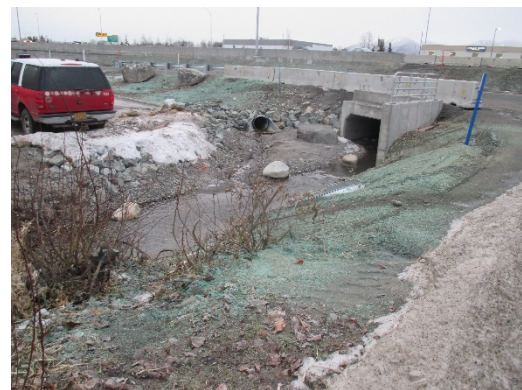
South Fork Little Campbell Creek box culvert outlet lacking down-slope sediment control measures/physical controls
